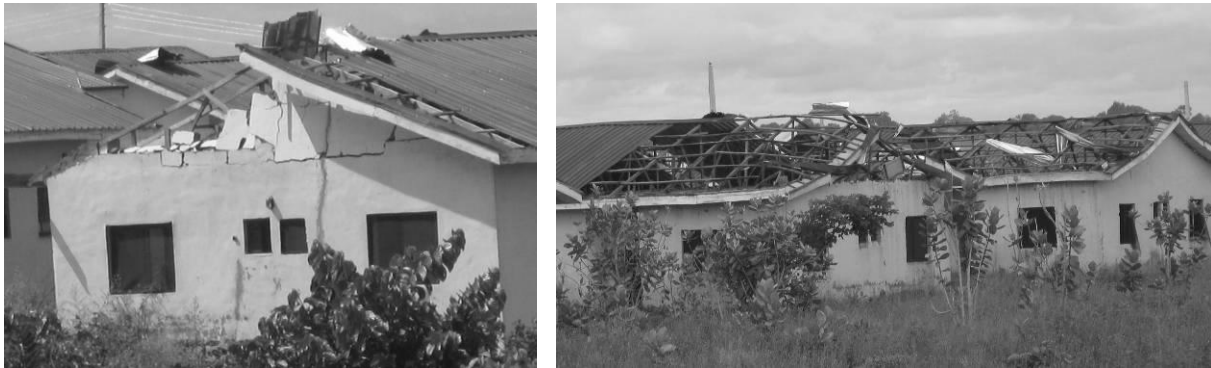
Fig 5: Views of the Talba housing estate depicting uniform pattern of material waste along the gable end owing to flawed roof design and poor building orientation. Source: Author's field work, 2011
