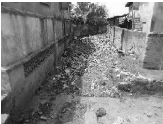
Plate 4: Refuse dumped inside drainage channels which hinders free flow of run-off Source: Field Survey, 2011
