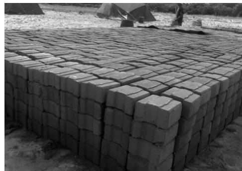
Pic 2: The Hydraform blocks ready for the first building. Source: Malaika Kids UK website.
